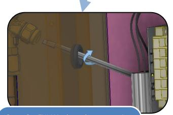
Step 3: FULLY shut the expansion valve (turn the screwdriver clockwise). Check the position of the tip of the screwdriver (to give it the right number of turns for correct expansion valve adjustment)
