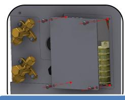
Step 1: Unscrew and remove the electrical access plate of the outdoor unit.
